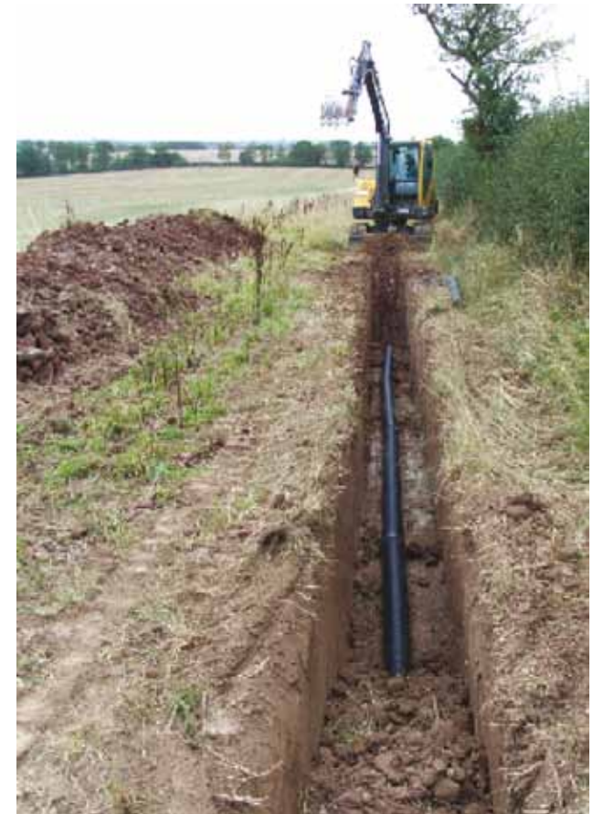
Laying the 550 metres of conduit.
