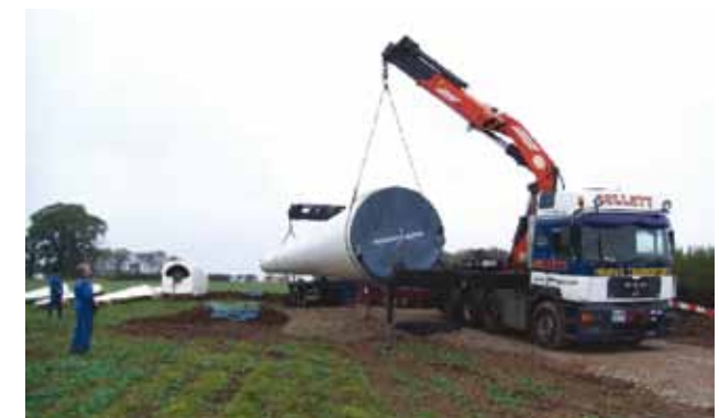
Two cranes needed for the tower.
