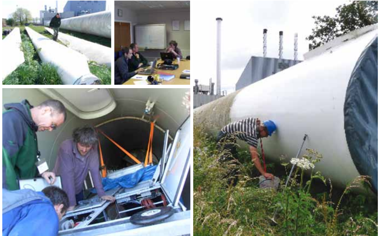
Clockwise from left: First site of Turbine. Meeting at INEOS. Cleaning the Turbine. Inside the base of the tower.
